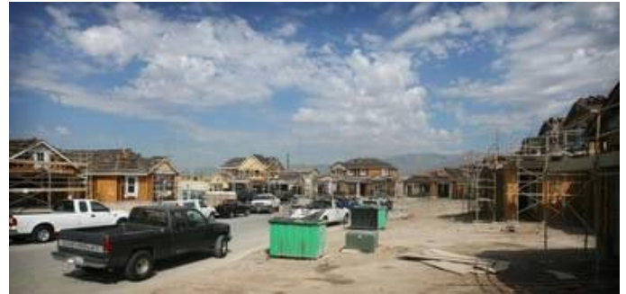
Construction in City of Eastvale
